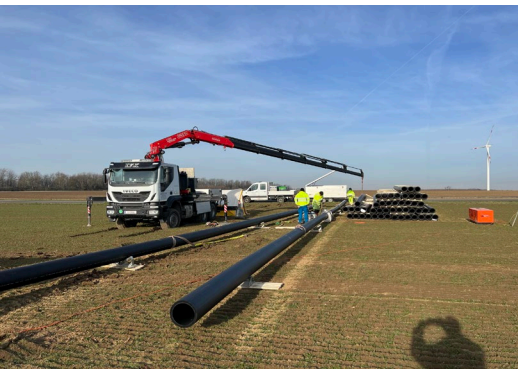
Image, left: using the ploughing method, even long pipe sections can be laid in the shortest possible time and with significantly less environmental impact; image, centre: the ploughshare with the displacer is the so-called leading edge when it comes to underground installation; image, right: to create the extensive piping system, several pipe sections with up to 60 pipes were interconnected using the heated-tool butt welding method
