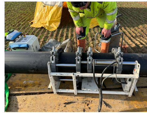
Image, left: using the ploughing method, even long pipe sections can be laid in the shortest possible time and with significantly less environmental impact; image, centre: the ploughshare with the displacer is the so-called leading edge when it comes to underground installation; image, right: to create the extensive piping system, several pipe sections with up to 60 pipes were interconnected using the heated-tool butt welding method
