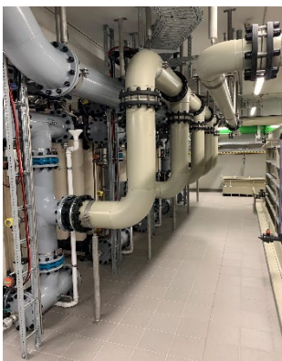
Top left: ventilation and deaeration line, neutralisation tank Bottom left: sludge water line, ultrafiltration unit Right: circulation line, neutralisation tank
