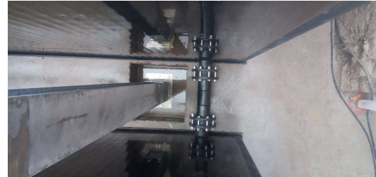
From left to right: Installing the rainwater storage tanks on site with a crane; assembly of the joints and connections to the overall rainwater utilisation system; connection of the two rainwater storage tanks by means of a DN200 overflow pipe
