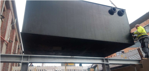
From left to right: Installing the rainwater storage tanks on site with a crane; assembly of the joints and connections to the overall rainwater utilisation system; connection of the two rainwater storage tanks by means of a DN200 overflow pipe
