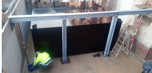
From left to right: Installing the rainwater storage tanks on site with a crane; assembly of the joints and connections to the overall rainwater utilisation system; connection of the two rainwater storage tanks by means of a DN200 overflow pipe
